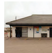
Reusing existing buildings is the premise of the approach of the project which is best practice in terms of sustainability
